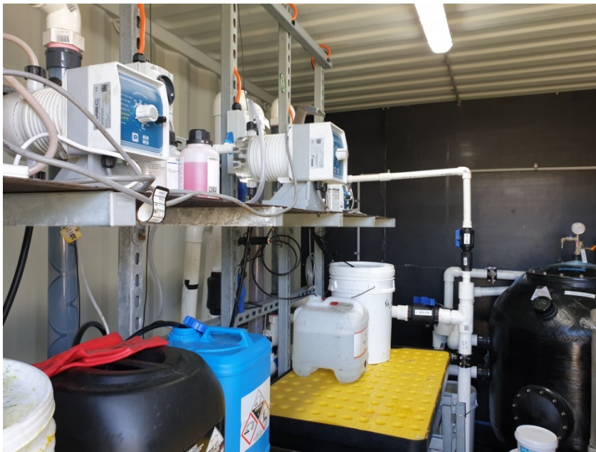
Figure 6 Insite PFAS Treatment Trial at Fire Training Ground
