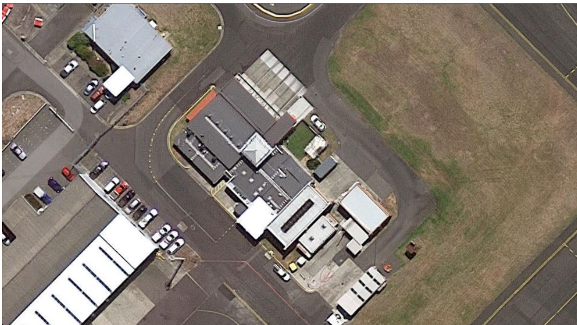
Figure 7 Field trial location for X55 at the Fire Station Building
