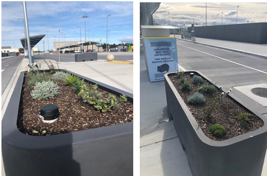
Figure 4 Forecourt Wicking Bed Planter Boxes
