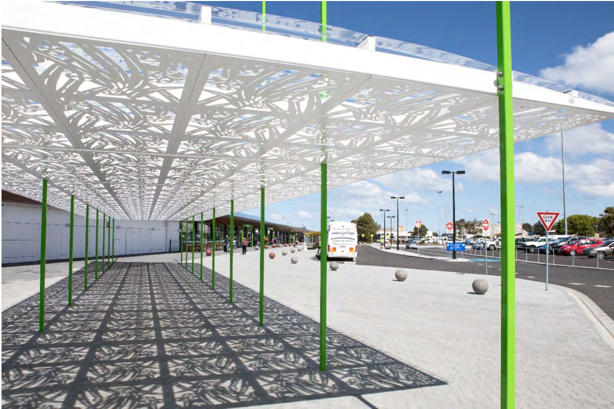
Figures 5 and 5.1 Existing Terminal Building Forecourt and Parking Subject to Terminal Expansion Works
